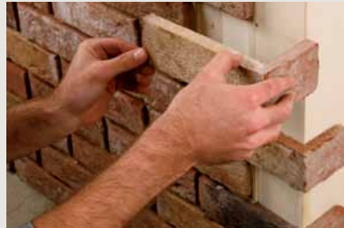
5 Applying the connecting strips
