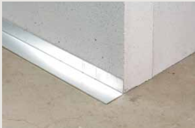
1 Placing the starting guide post
