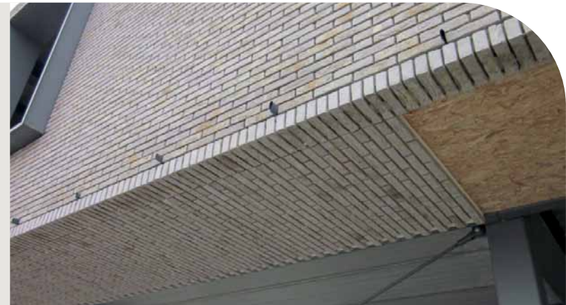
Ceiling finishing with facing bricks
