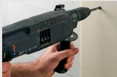
2 Placing the corners
